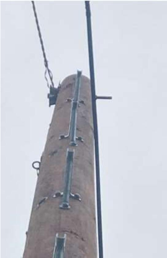
**3.3 Mid Span contact between newly erected CP Wire and BT Dropwire.**
